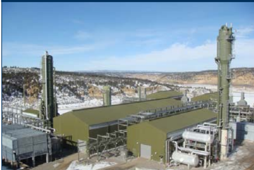
Natural gas processing plant
